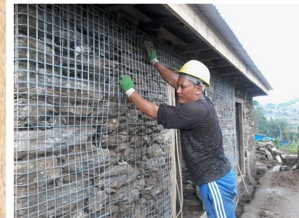
Photo caption: Glimpses of Retrofit training conducted in Dolakha. 25 days Retrofit training intends to retrofit an existing private house with cracks or not at all and develop 6 masons with the retrofit skills in their hand.
