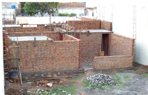
Construction sequence of confined masonry
