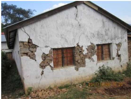
Diagonal cracks
