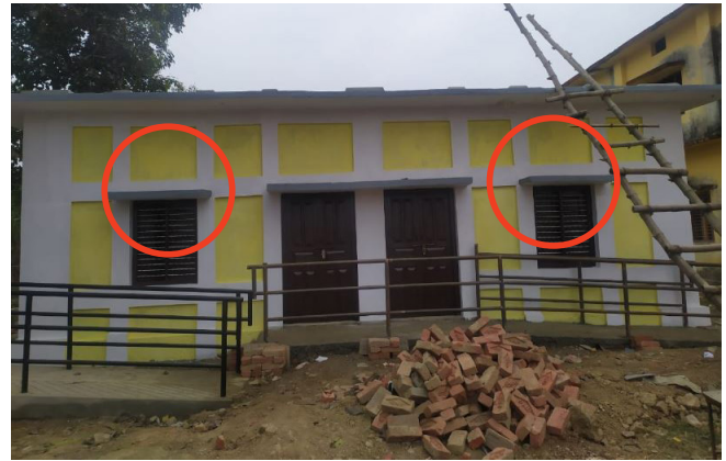
Openings closed after retrofitting
