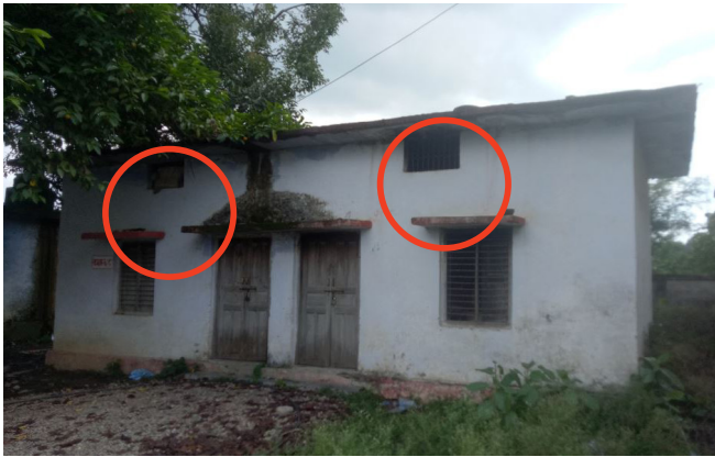
Existing openings prior to retrofitting
