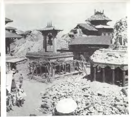
The destruction that occurred during the earthquake in Bhaktapur around the Thapliya Hill
