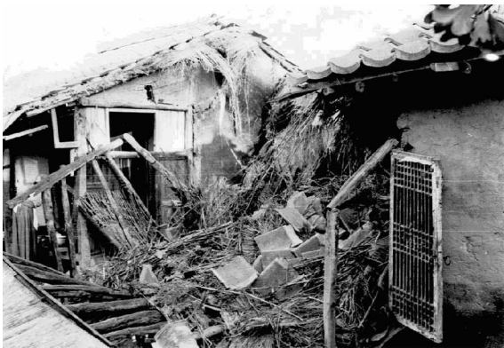
Figure 2. Collapse of house during the 1978 Hongsung earthquake
