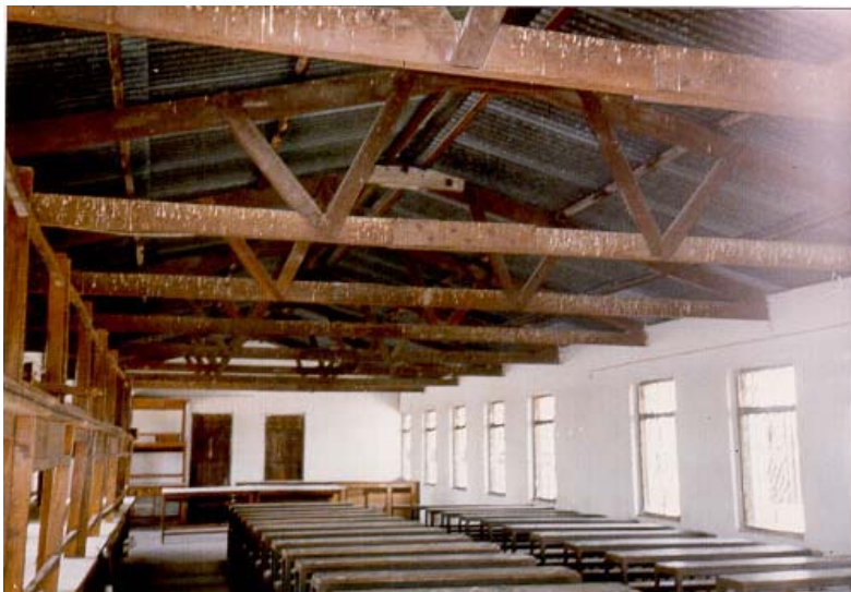
Photograph 4.7: CGI sheet laid over Timber truss. [NSET-Nepal's Archive]
