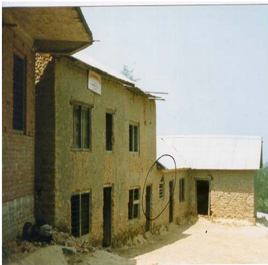
Single pitched CGI Sheet roof on one story stone and sun dried brick mixed wall in mud mortar. Floor is constructed of timber.
