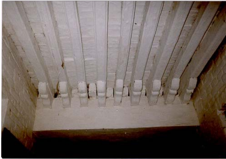
Photograph 4.6: Floor constructed with earth laid on brick supported by timber joist. [NSET-Nepal's Archive]
