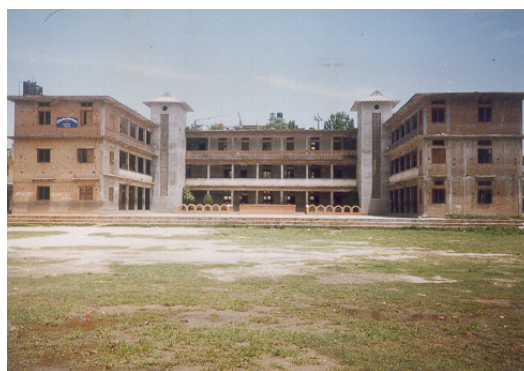
RC floor and roof slabs supported by fired brick wall. All walls of first story and partly of second story are in mud mortar and rest in cement mortar
