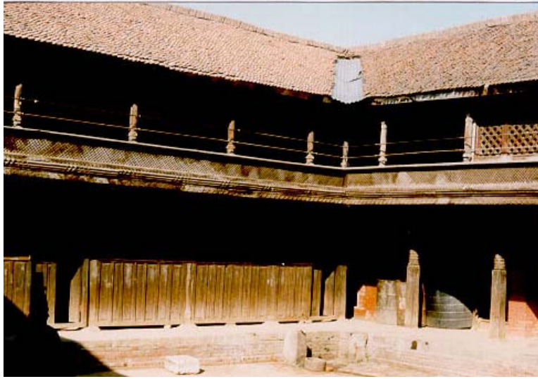
Photograph 4.8: Jhingati (clay roofing tiles) laid over timber structure. [NSET-Nepal's Archive]
