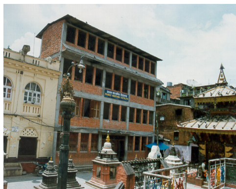
Multistoried RC framed building with CGI sheet roof and RC floor Slabs.
