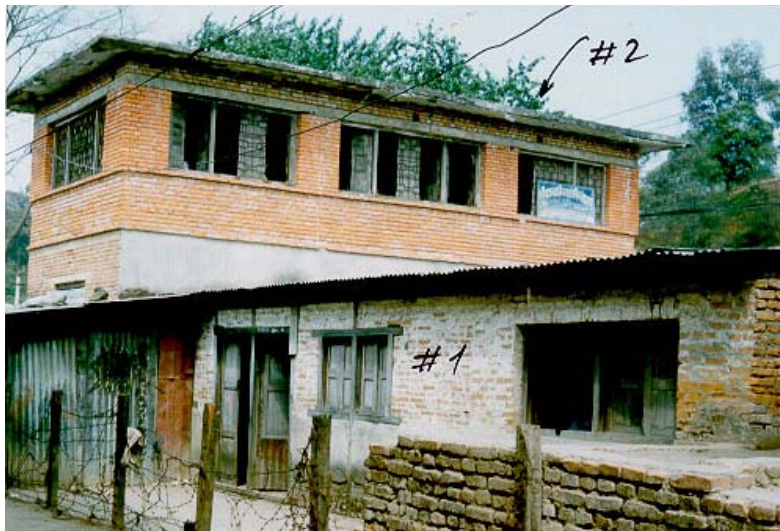
Photograph 4.10: No lintels at all over openings. [NSET-Nepal's Archive]
