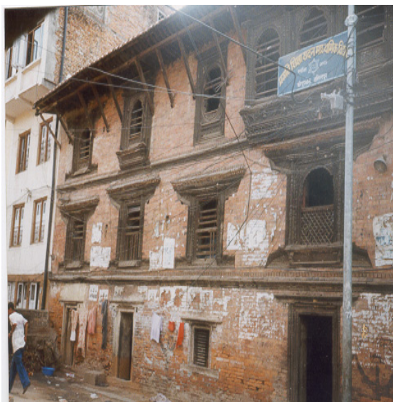
Pragti Siksha Sadan, Kupondole, Walls in fired brick in mud mortar, timber floor, Clay tile roof on Timber structure medieval architecture, Constructed much before (2000 B.S.)
