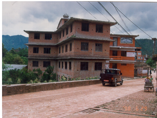
A four –story masonry building with RC roof and floor slab. Mind first two stories are in brick in mud mortar where as upper one are in brick in cement mortar.
