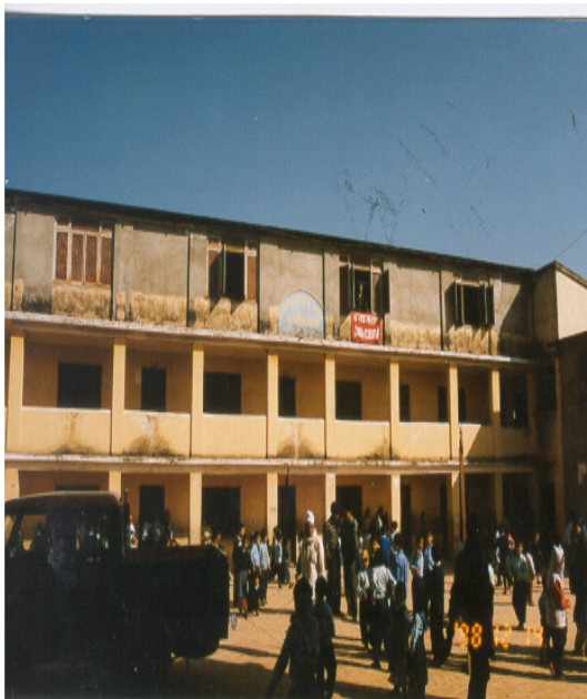
A three- story masonry building in brick in cement mortar with flexible roof.
