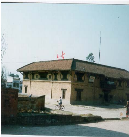
Courtyard type building, walls in brick in cement mortar, timber floor and tile roof on timber structure (const. By Bhaktapur Dev. Project)
