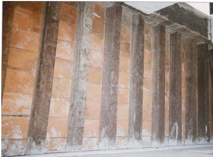
Photograph 4.5: Floor constructed of plain concrete laid over brick supported by timber joist. [NSET-Nepal's Archive]
