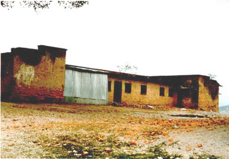
Photograph 4.18: Lack of maintenance leading school building to severe deterioration. [NSET-Nepal's Archive]
