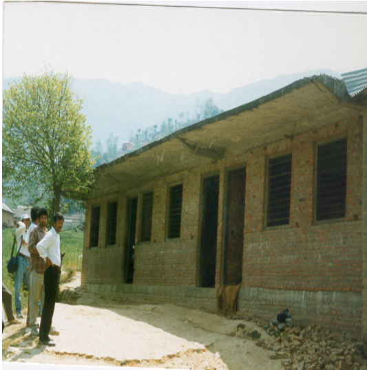
Single storied RC slab roof on brick in cement mortar wall.
