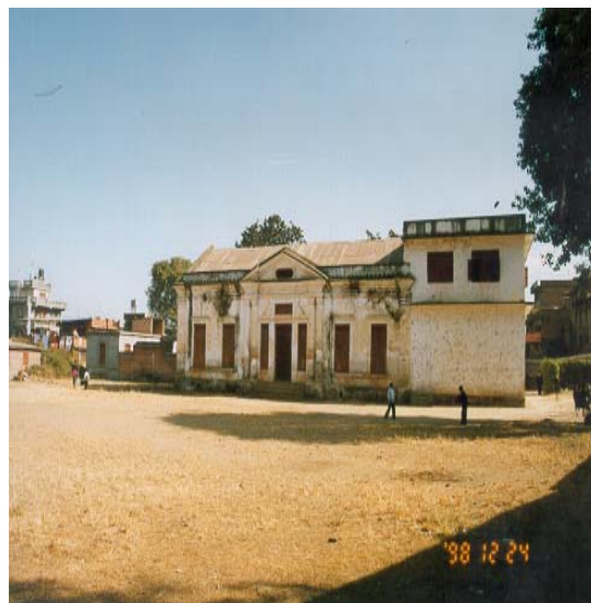
A Rana Era Victorian style one story school building. Walls brick in lime, CGI sheet roof on timber structure ( Constd. Befor e 2000 B.S.)
