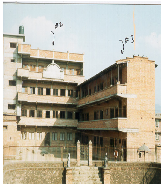
Multistoried RC framed building with RC floor and roof slabs. Adjacent is three storied brick building in cement mortar, RC floor slabs and CGI Sheet roof.
