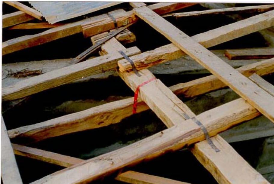
Photograph 5.1: Improving the roof integrity by nailing and strapping. [NSET-Nepal's Archive]
