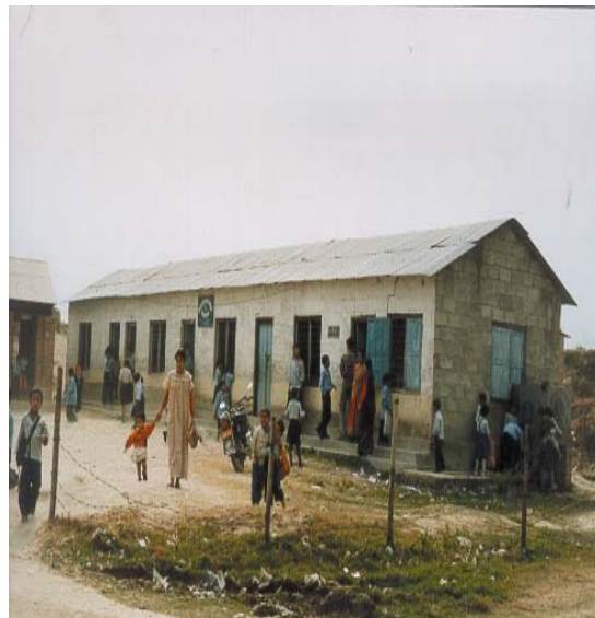
A masonry school building shed in hollow concrete block in cement mortar, mind the cracks.
