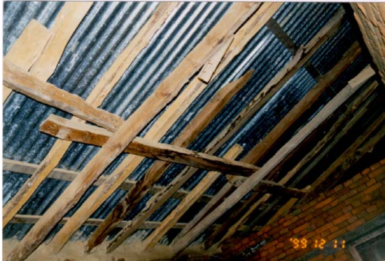
Photograph 4.12: Loose fit timber roof structure. [NSET-Nepal's Archive]
