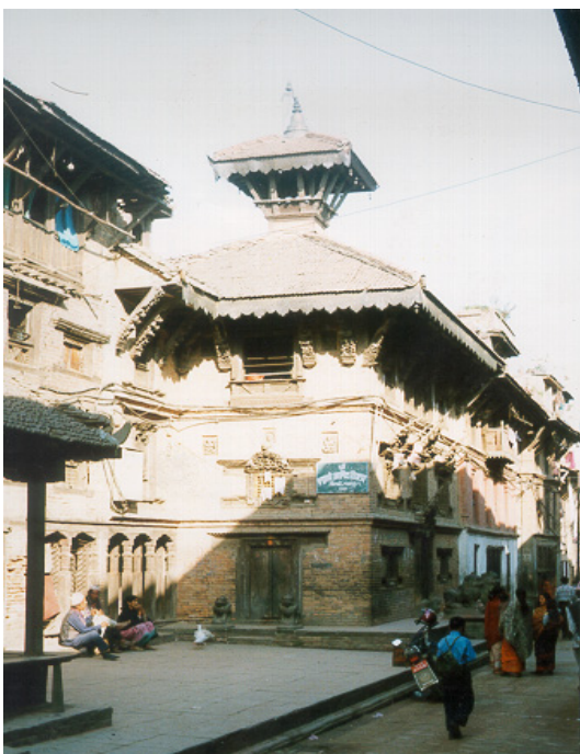
A school building in dense urban area. Clay tile roof and Timber floor resting on fired brick in cement mortar (constd. By Bhaktapur Development Project)
