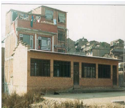
CGI Sheet roof on brick in mud mortar wall.
