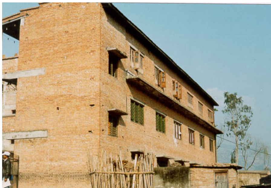
Photograph 4.2: Timber lintel in masonry building. [NSET-Nepal's Archive]
