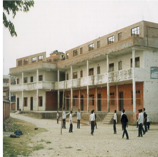
RC framed building under vertical extension.
