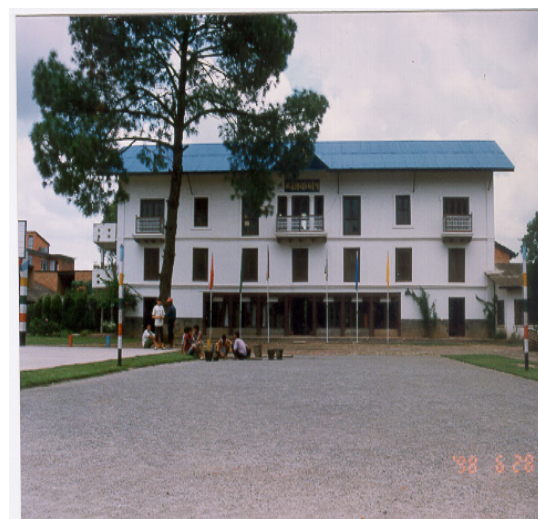
Multistoried RC framed building with RC floor and roof slabs. Adjacent is three storied brick building in cement mortar, RC floor slabs and CGI Sheet roof.
