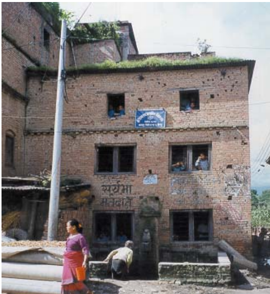
CGI Sheet roof on brick in mud mortar wall.
