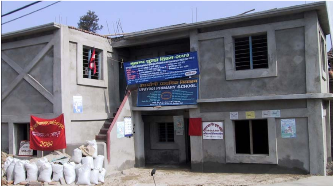
Photograph 5.2: Splint and bandage technique for retrofitting masonry building. [NSET-Nepal's Archive]
