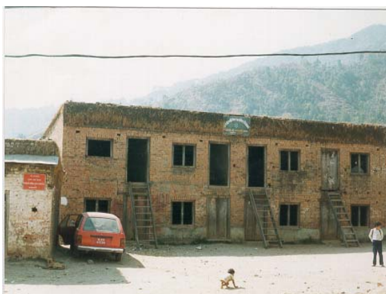
Single Pitched CGI Sheet roof and timber floor in red brick in mud mortar.
