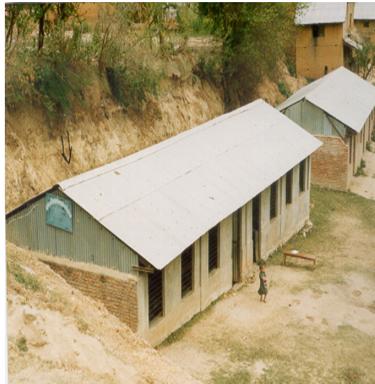
Earthquake block with masonry infill in brick cement mortar.
