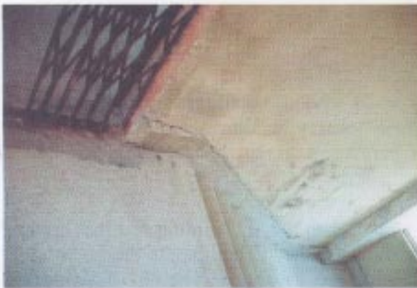
Cracks in pounding area between the "wedge" and the "L" building. Left: Top storey. Right: First storey.
