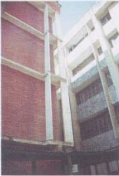
"L" building: Left: Masonry or RC blocks can fall down and injure people during a MMI = VI-VII earthquake. Middle and Right: Short columns will be able to trigger the building and lead to fragile-collapsing-mechanism (pancake failure) during a MMI = VII earthquake.
