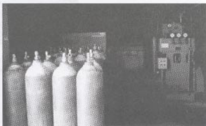
Left: Oxygen cylinders in a storage area. Right: Oxygen cylinders in the central oxygen room. To reduce non-structural vulnerability it is necessary to keep slender equipment, harmful to people, well-fitted and restrained against overturning.
