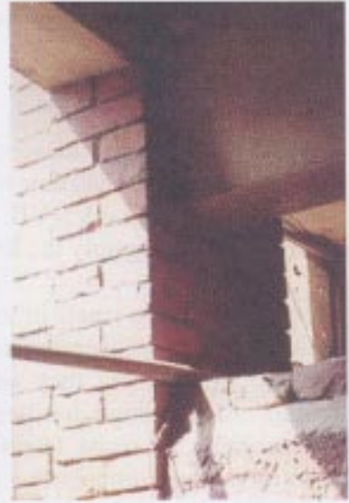
"L" building: Left: Masonry or RC blocks can fall down and injure people during a MMI = VI-VII earthquake. Middle and Right: Short columns will be able to trigger the building and lead to fragile-collapsing-mechanism (pancake failure) during a MMI = VII earthquake.
