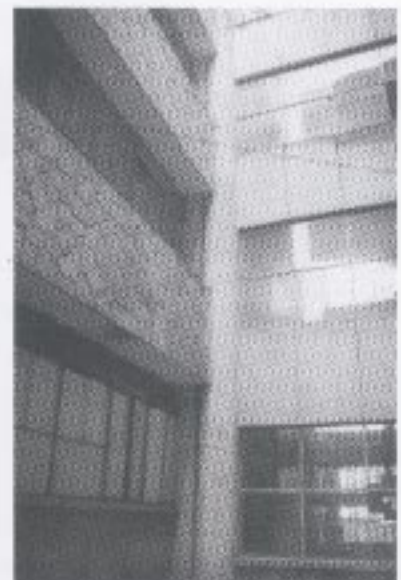
"New" buildings. Left: Seismic joint of small size in the main building facing Kanti Path. Middle: Diaphragm discontinuity in one of the three structures composing the main new building. Right: Masonry parapets rigidly connect the new buildings where a seismic joint was designed.
