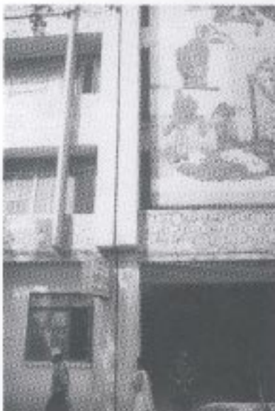
"New" buildings. Left: Seismic joint of small size in the main building facing Kanti Path. Middle: Diaphragm discontinuity in one of the three structures composing the main new building. Right: Masonry parapets rigidly connect the new buildings where a seismic joint was designed.
