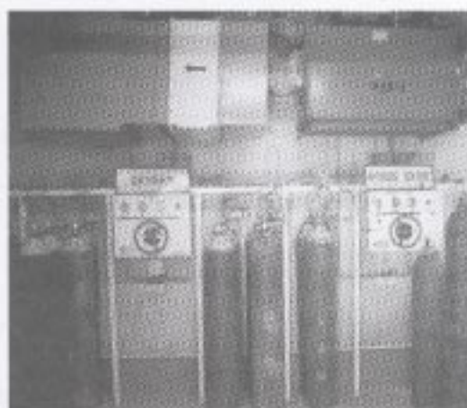
Central oxygen room. Left: Oxygen plant. Maintenance is very good for local standards. Right: Oxygen cylinders being refilled. The lateral stability of such cylinders should be improved by using devices designed to fit the cylinders to the ground while they are refilled.
