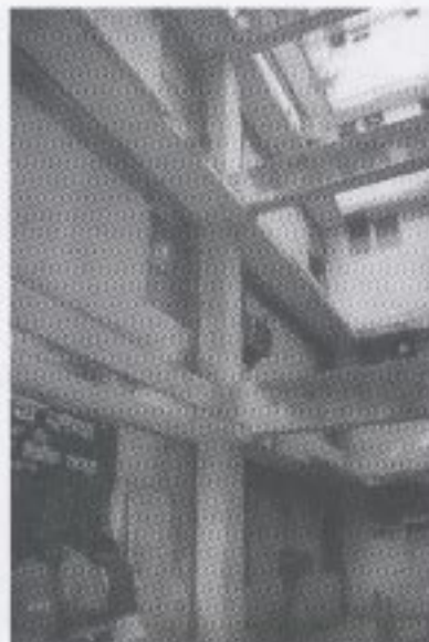
"New" buildings. Left: Seismic joint of small size in the main building facing Kanti Path. Middle: Diaphragm discontinuity in one of the three structures composing the main new building. Right: Masonry parapets rigidly connect the new buildings where a seismic joint was designed.
