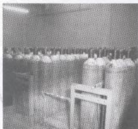
Left: Oxygen cylinders in a storage area. Right: Oxygen cylinders in the central oxygen room. To reduce non-structural vulnerability it is necessary to keep slender equipment, harmful to people, well-fitted and restrained against overturning.
