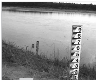
Figure 4.3: Water-level-gauge installed at the river bank
