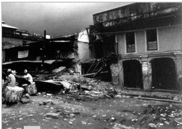
Figure 3.3: Building damage in Naya Bazar of Dharan
