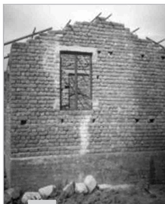
Figure 3.13: Detached toilet blocks for the houses
