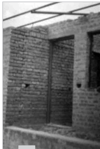
Figure 3.10: Brick building under construction
