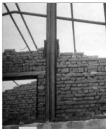
Figure 3.11: Pre Cast RCC lintel above the opening
