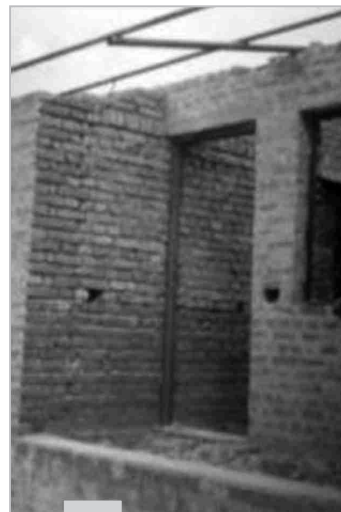
Figure 3.10: Brick building under construction
