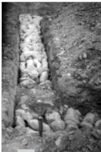
Figure 3.8: Stone Masonry in Foundation
