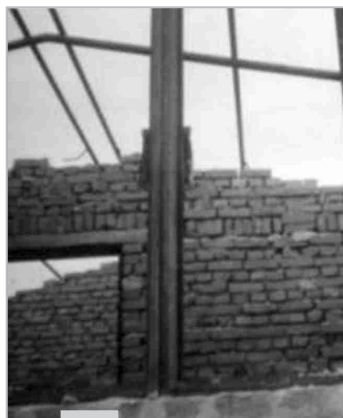
Figure 3.11: Pre Cast RCC lintel above the opening
