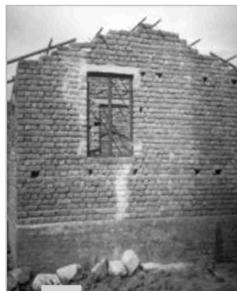
Figure 3.13: Detached toilet blocks for the houses
