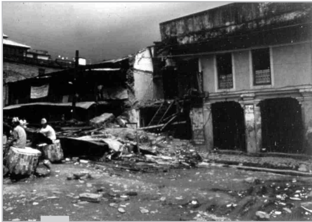
Figure 3.3: Building damage in Naya Bazar of Dharan
