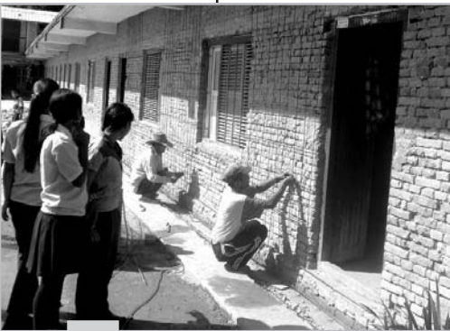
Figure 4.17: Students observing the retrofitting work in one of the selected school
