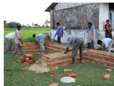
Trainees making masonry full scale model
