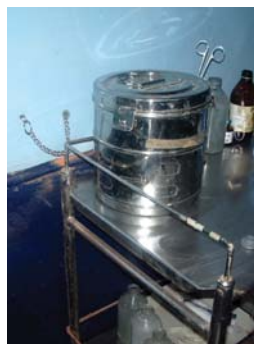
Trolley being hooked on a wall as a part of non-structural mitigation
