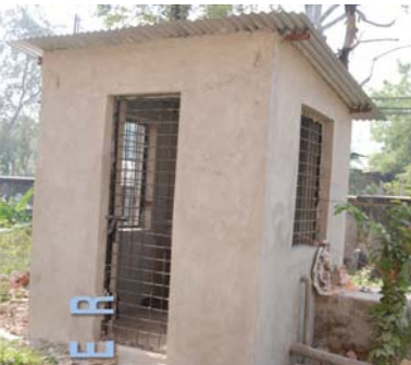
Earthquake resistant pump house
