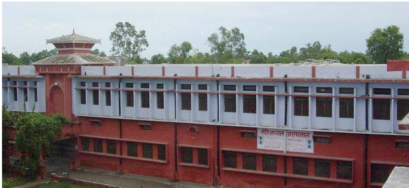
A step towards hospital safety: Bheri Zonal Hospital
