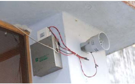
Siren being installed on hospital premise
