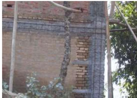
Fig. 81 : Stitching of transverse walls
