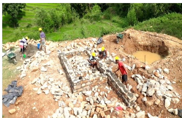
Masonry work in disaster-friendly toilets construction
