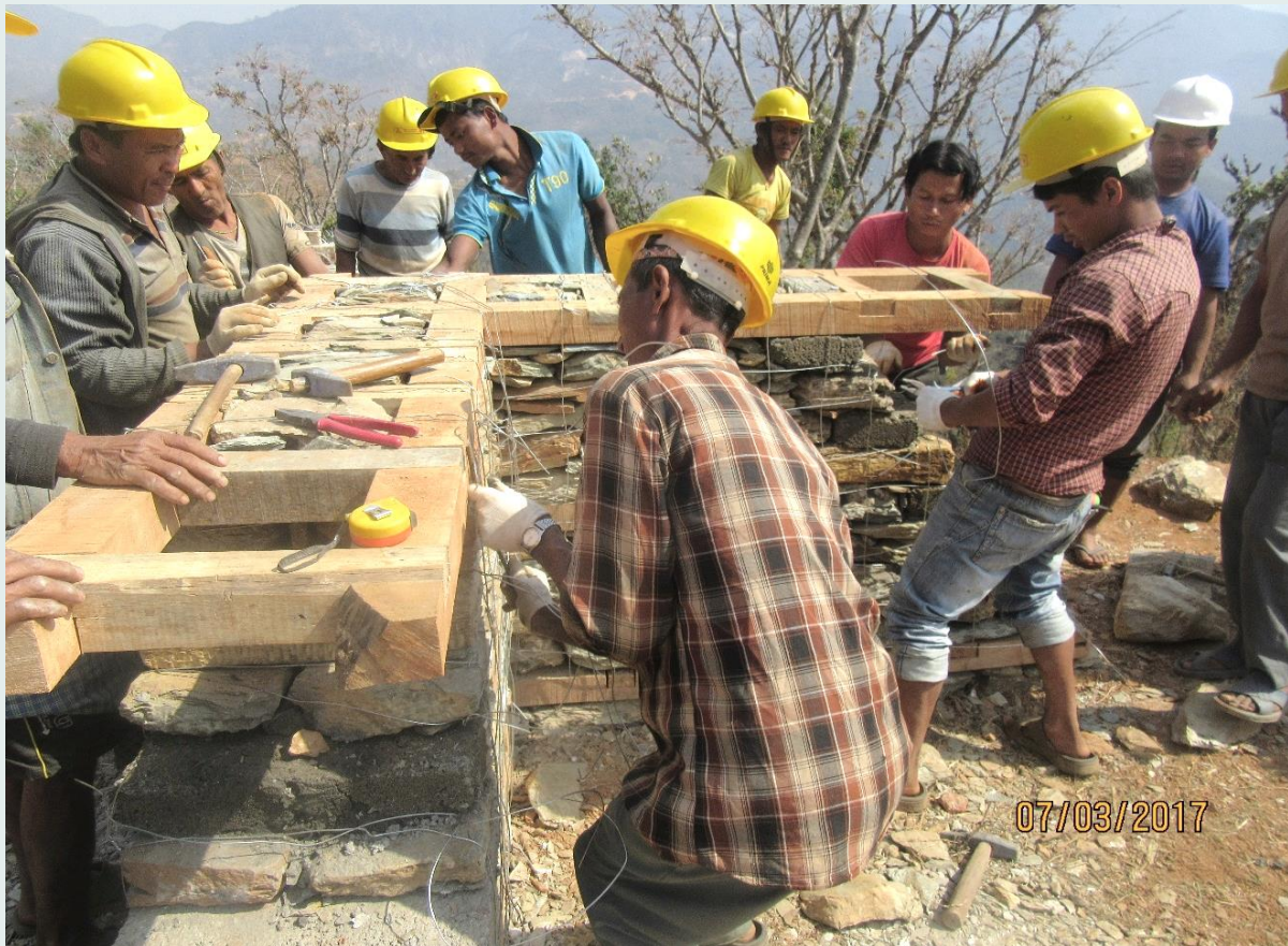
Participants working on construction of wooden bands during hands on practical exercise of rural mason training in Dhading.
