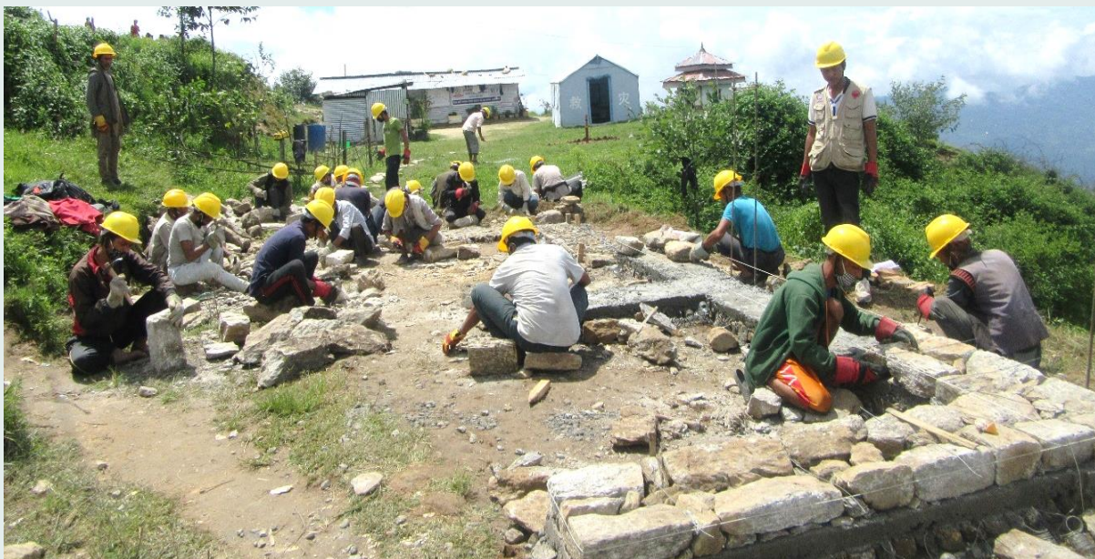
Training participants working together in construction of stone masonry walls using earthquake resistant construction techniques in Dolakha. Participants constructed a small scale model of masonry walls to apply hands on practice of the techniques of construction under close supervision of instructors.
