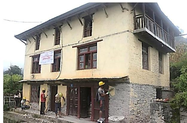
Relying on the curricula, retrofit training have been conducted through which demonstration models have been installed in the communities. The primary work during the period (July-Sept 2019) was to implement retrofit in masonry buildings as did in previous months. In this period, 16 houses in program areas were retrofitted as part of mason trainings, with two houses still under construction due to obstructions in road and house owner limitations during festivals.
