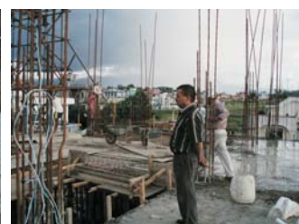
First floor slab casting
