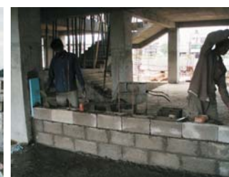
Polystyrene in between the column and infill wall
