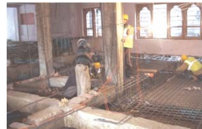
Work in Progress, placing reinforcement bars on raft, beam, column and shear walls in Thimpu
