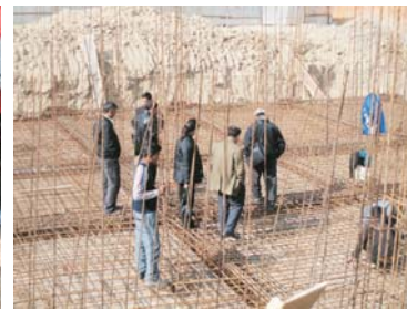
Basement Slab Reinforcement Checking
