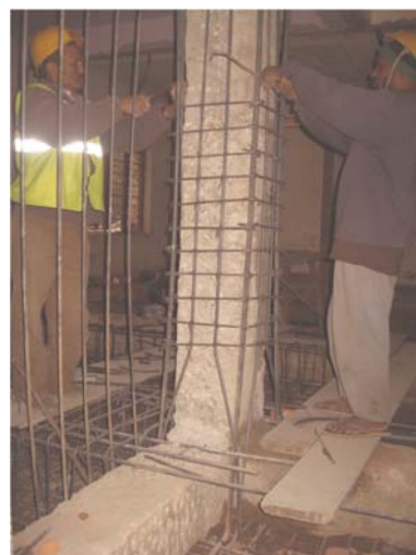
Jacking of the Column for earthquake-resistant building in Thimpu
