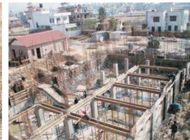
Basement columns construction
