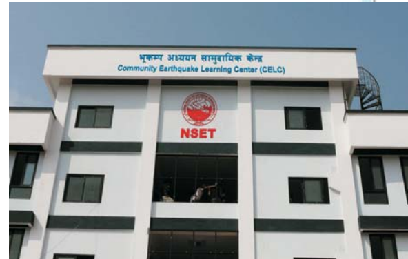
CELC Building at Bhainsepati
