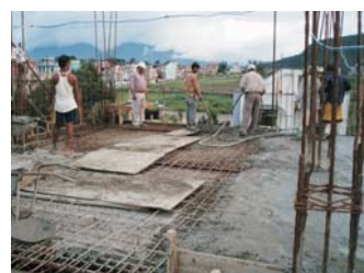
Concreting for second floor slab
