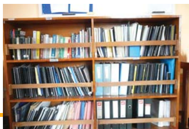
Non-structural Mitigation: Wooden straps in book rack Source: NSET
