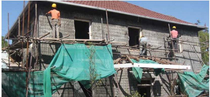
Retrofitting work in progress
