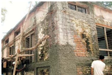
Retrofitting work in progress
